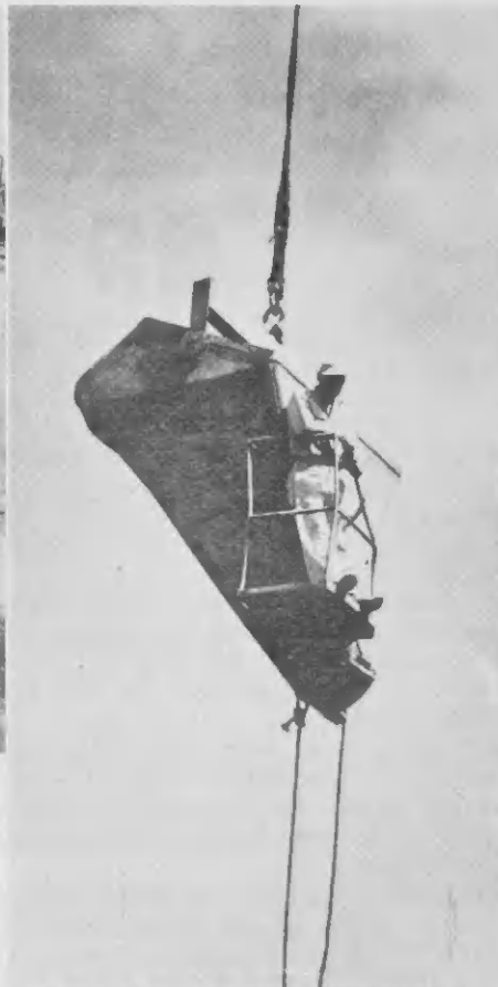
CORE SAMPLES were taken throughout the big pour. The hopper rider and vibrator man had unusual tasks.
